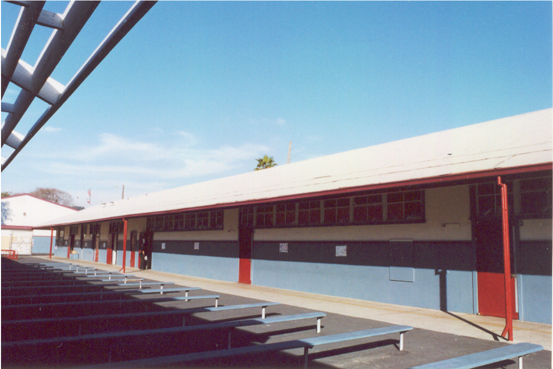
Figure 8: West Longitudinal Wall of Classroom Building (Typical)
