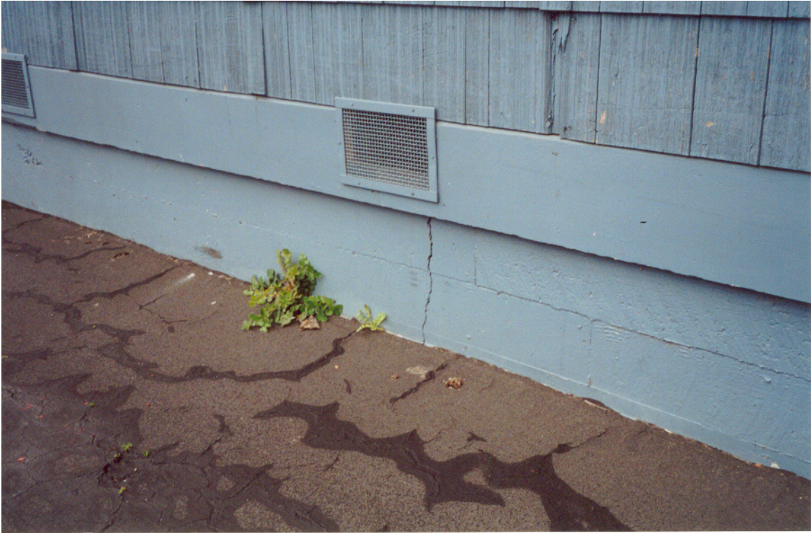
Figure 16: Cracking at Foundation of Permanent Portable Building
