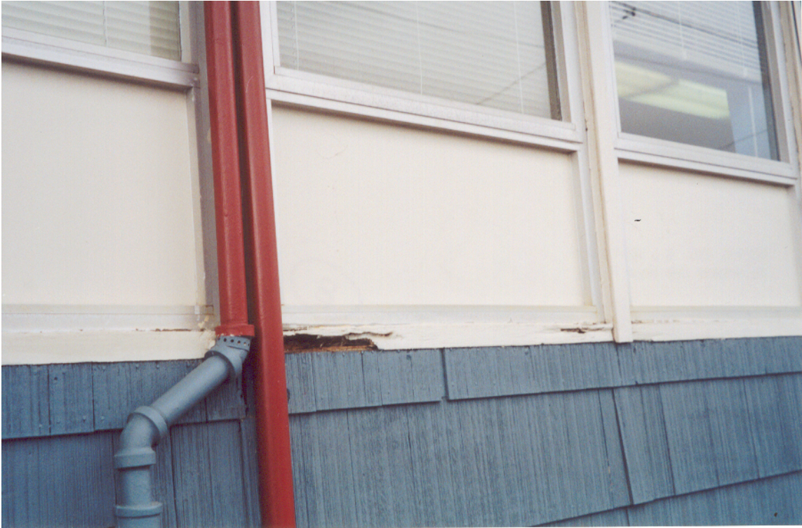
Figure 17: Dry Rot at Window of Permanent Portable Building
