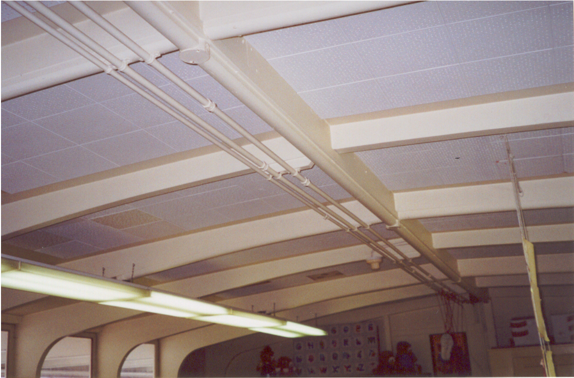
Figure 15: Interior of Permanent Portable Building
