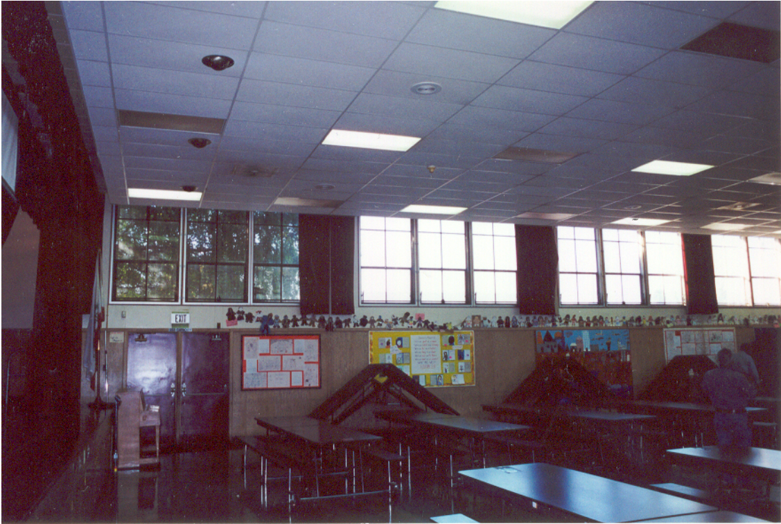
Figure 7: Interior of Multi-Purpose Building
