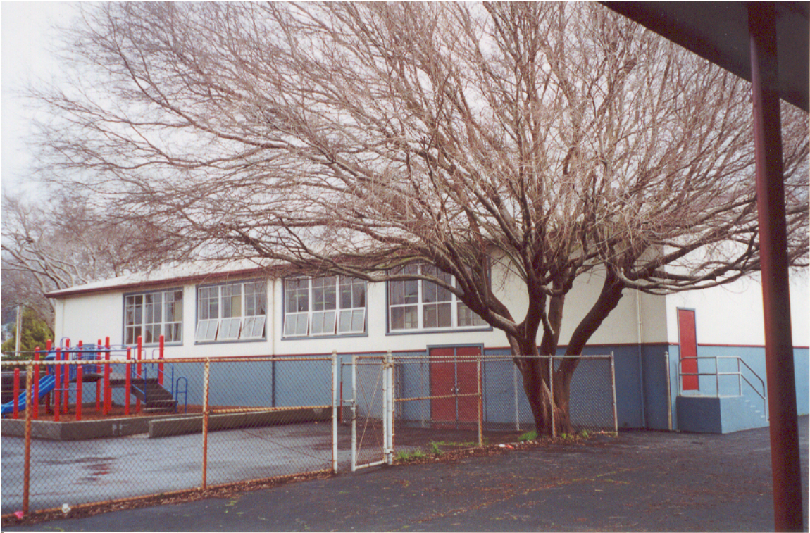
Figure 6: West Face of Multi-Purpose Building
