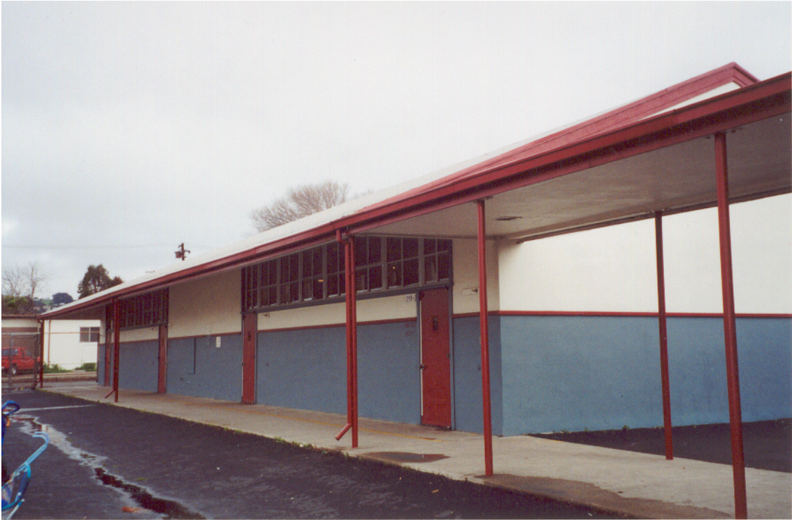
Figure 19: West Face of Kindergarten Building
