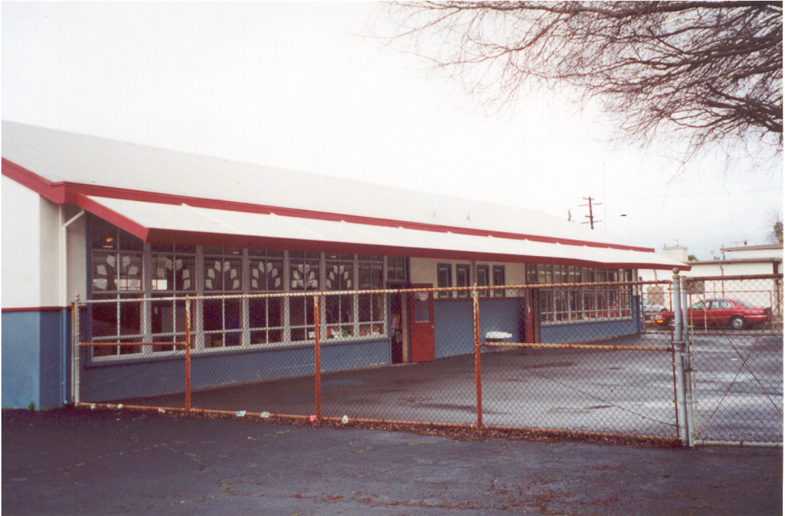
Figure 18: East Face of Kindergarten Building
