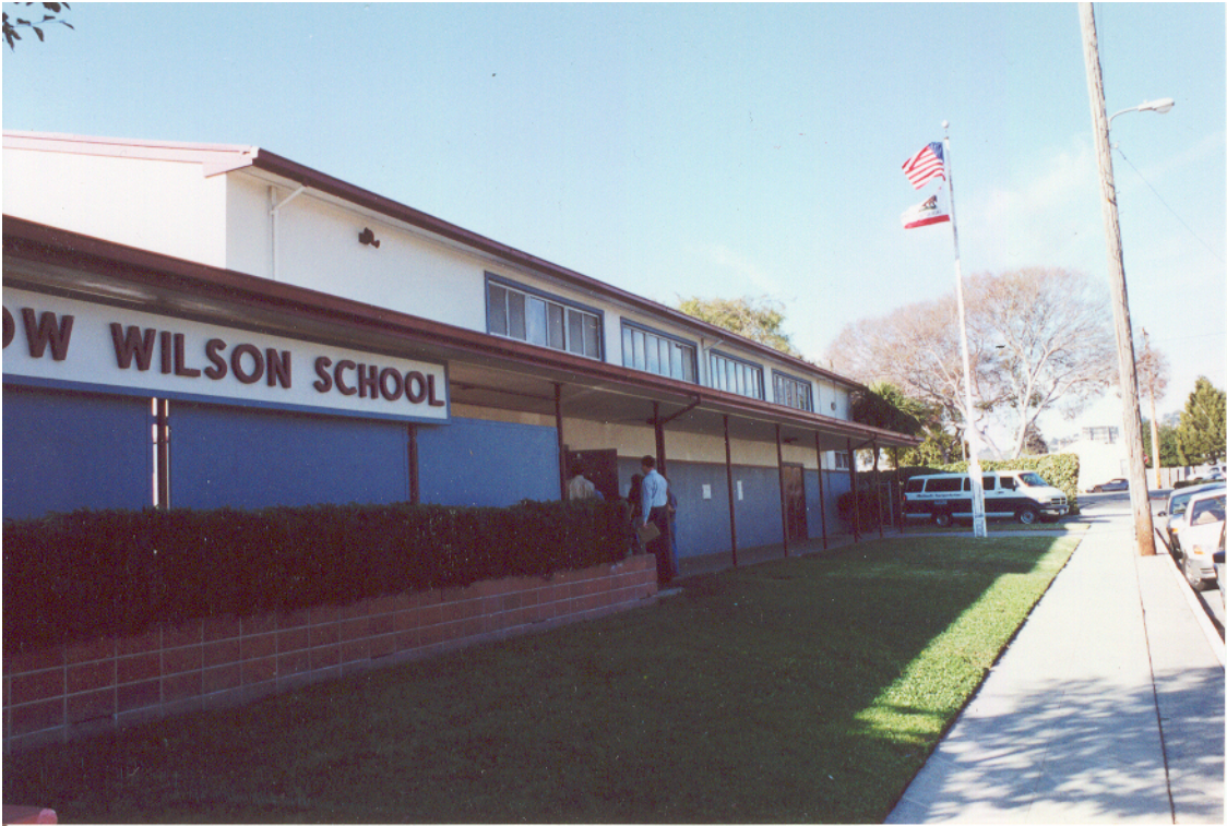
Figure 3: East Face of Multi-Purpose Building
