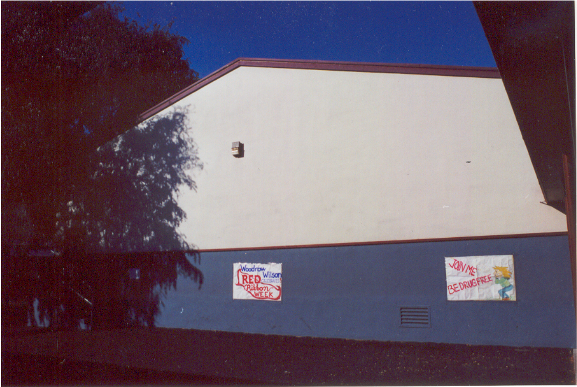
Figure 5: South Face of Multi-Purpose Building
